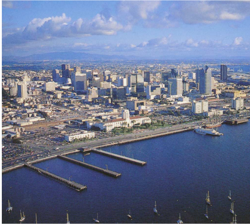
County Administration Building and Environs
